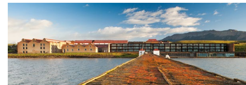
GENERAL VIEW FROM THE LOADING DOCK
